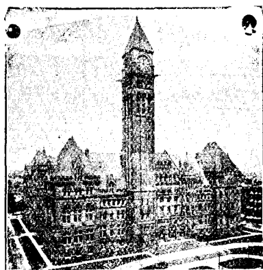
CITY HALL, TORONTO, CANADA. Hour Bell weighs 5 tons. Dials 20 ft. dia. The Largest Striking Clock in the NEW WORLD.
