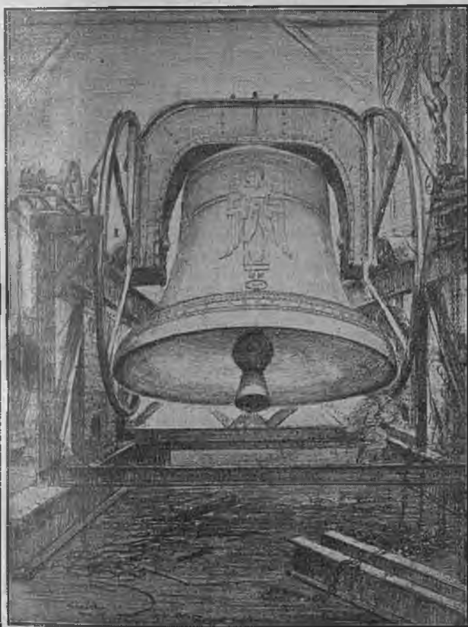
THE 18 1/2 TON RINGING BELL, the Bourdon of the Carillon of 64 Bells, about to be installed at RIVERSIDE CHURCH, New York, U.S.A
