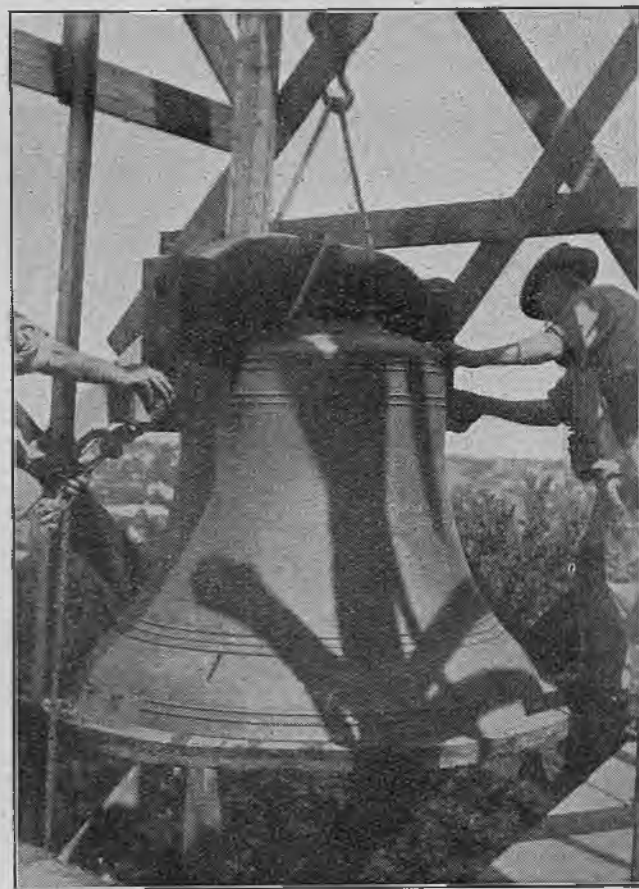
HOISTING THE TENOR BELL UP THE CATHEDRAL TOWER.
