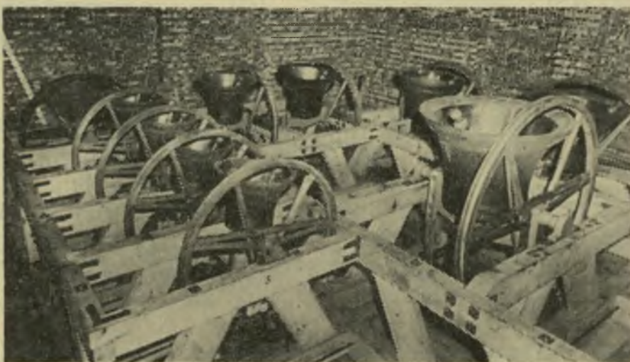
GUILDFORD CATHEDRAL BELLS. — The ten bells of Guildford Cathedral inside the brick tower. The frame is made of jarrah wood, which is noted for its hardness. When Messrs. Mears and Stainbank first visited the belfry they were very disturbed about the acoustics. The echo in the belfry was very alarming, but fortunately there has been time to have the concrete roof surfaced with acoustic material, which has eliminated the echo and thus enhanced the clarity of the bells.
