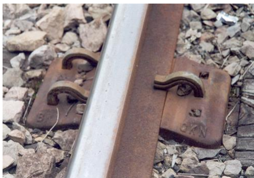
A BR1 cast iron baseplate. You won't need the rail unless you plan to run trains!
