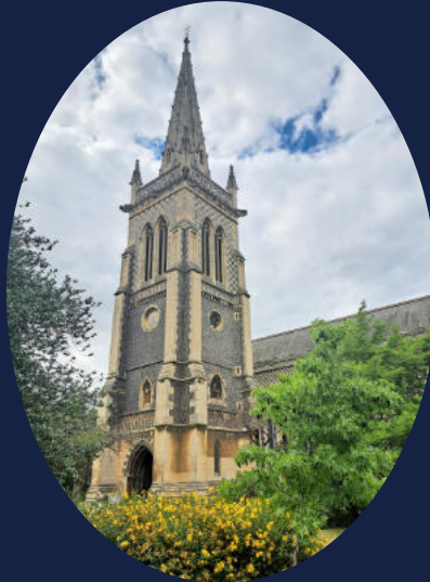
St Mary le Tower (12)
